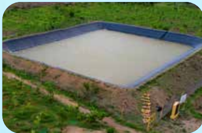
Water Pond Construction and Rainwater Harvesting Projects
